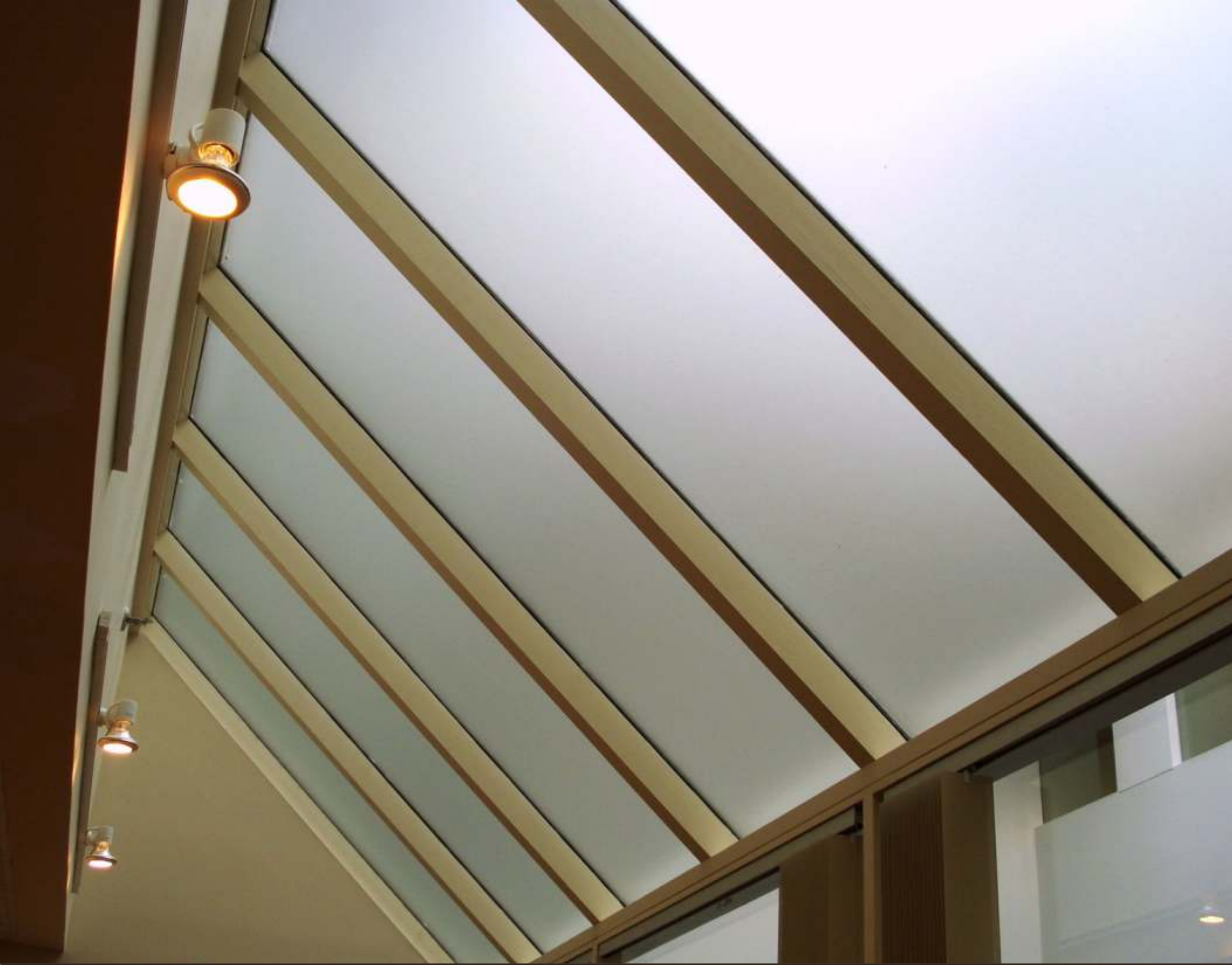
frosted film covering for overhead glass windows and skylight glass upper east side, new york city
