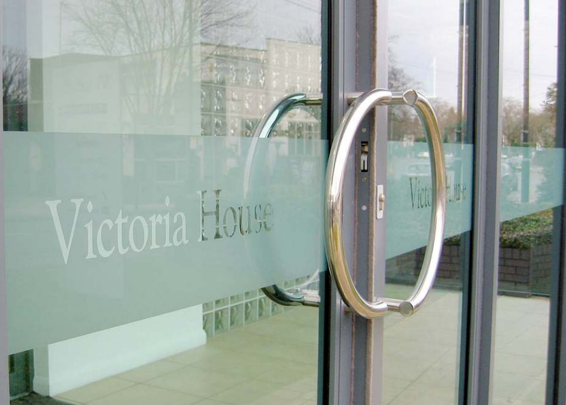
etched film distraction banding with logo knockout for storefront glass midtown east, new york city
