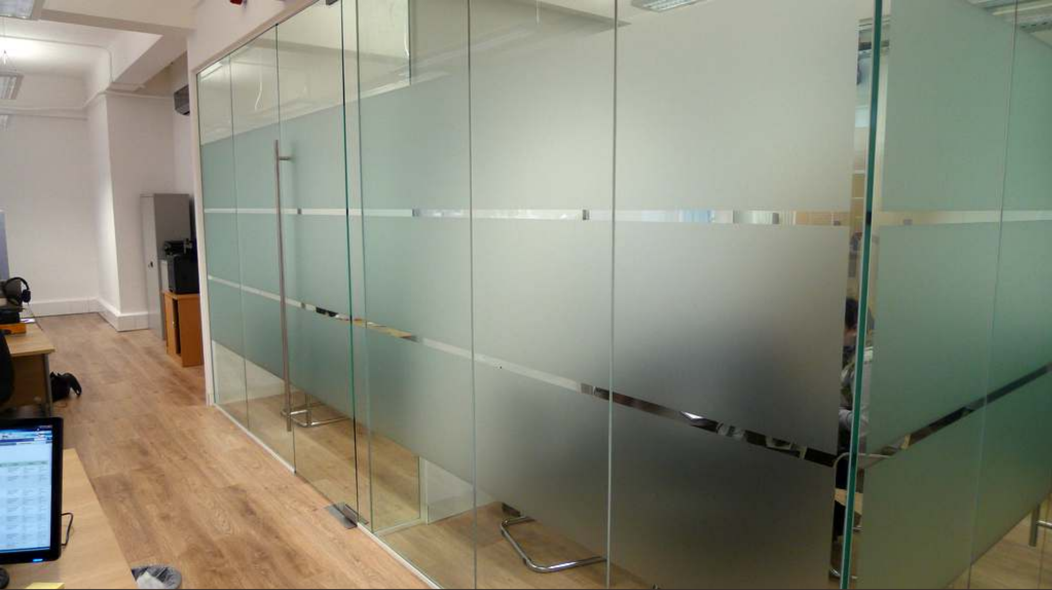
frosted banding on conference room glass panels with clear reveal soho, new york city
