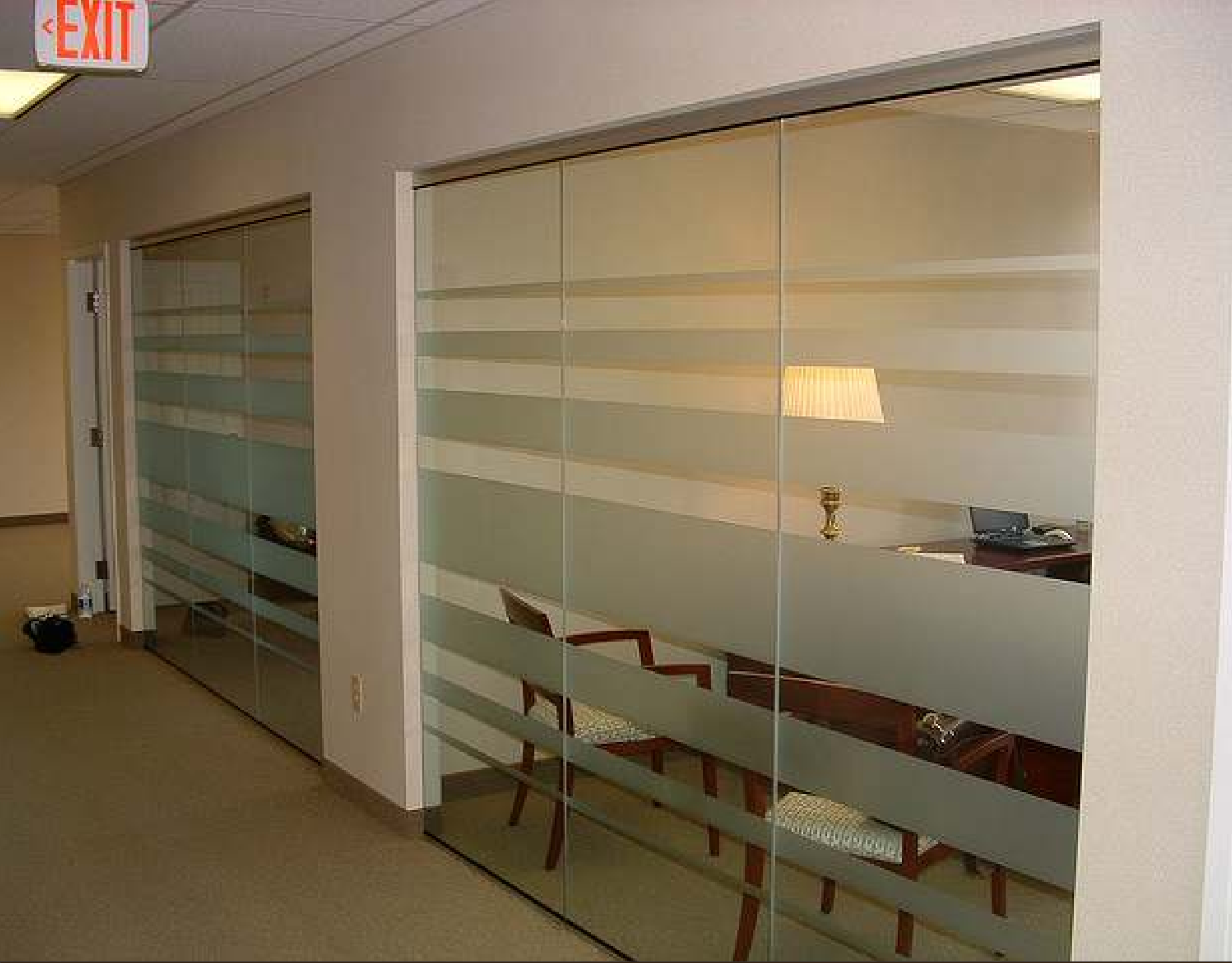
etched film privacy banding distraction marking for office rooms wall street, financial district, new york city
